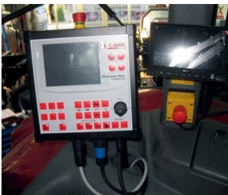
Process box and emergency stop for crane
